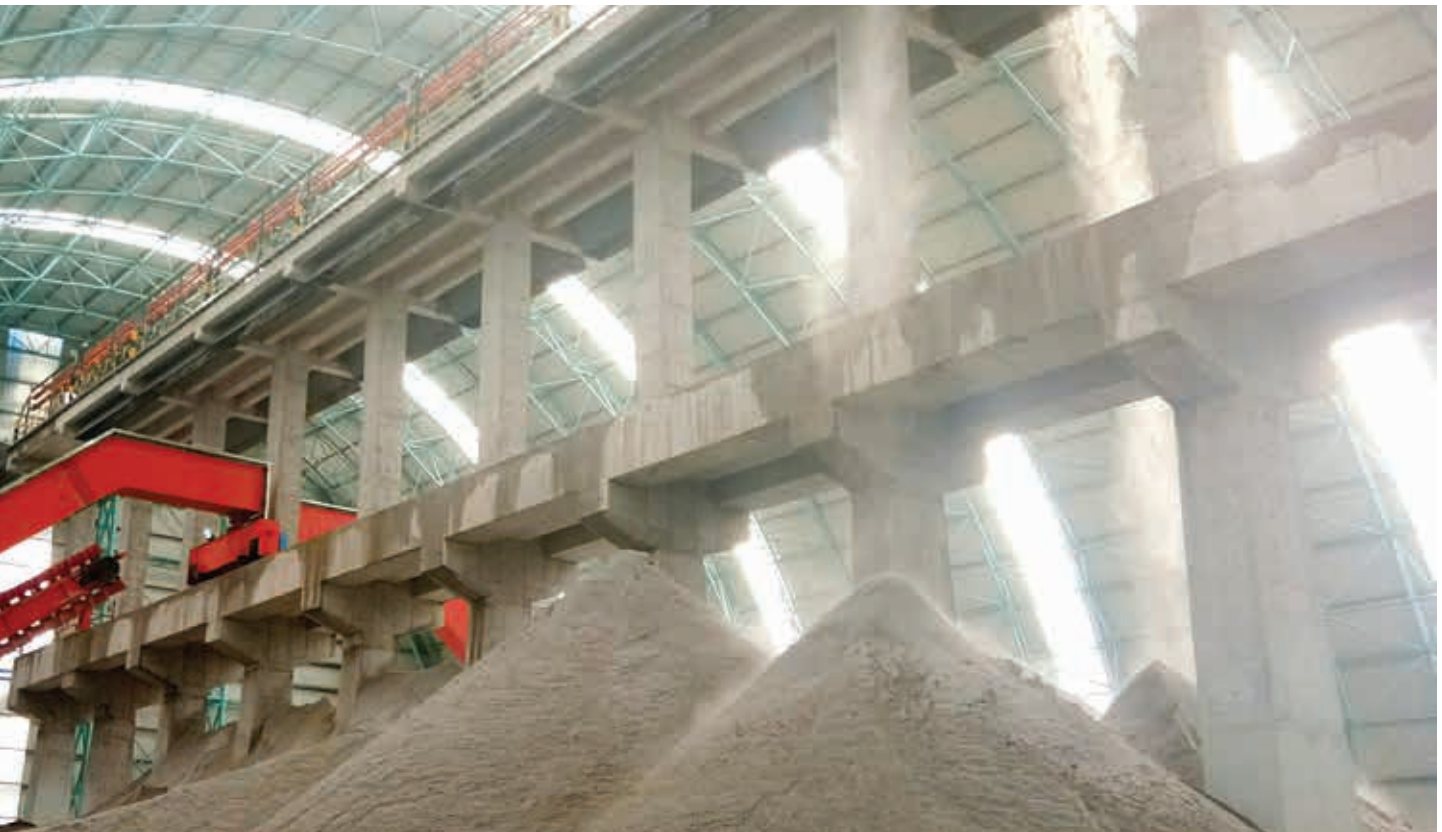
Photo: Slag receiving and storage in an enclosed system
