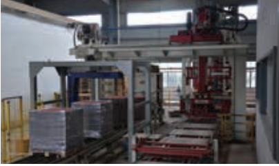
Wuxin Permeable Brick and Pavement Concrete Making Plant
