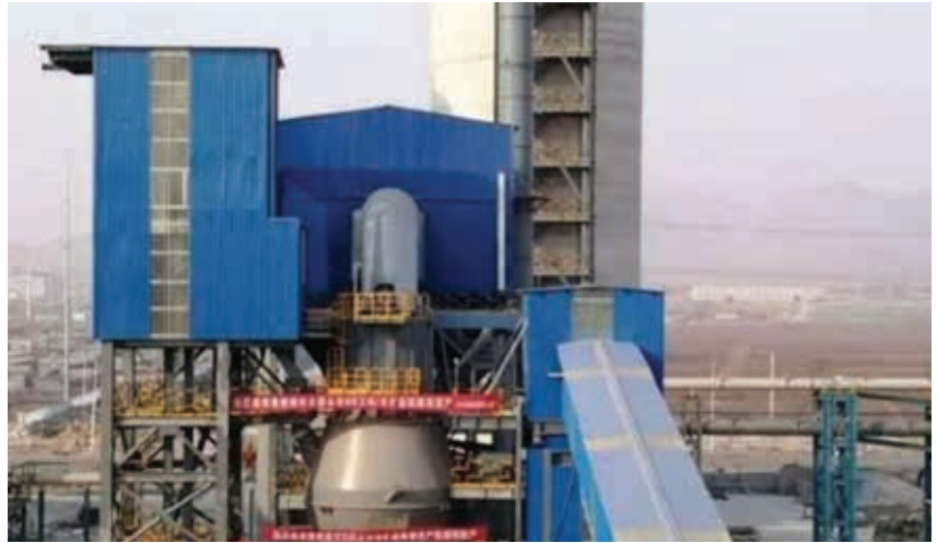
Photo: Rizhao Luxin GGBS Plant's Vertical Roller Mill ("VRM")
