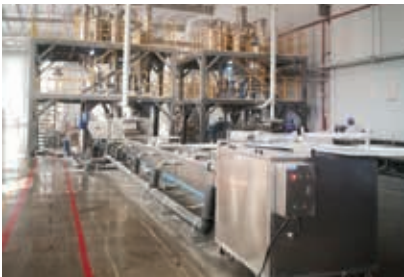
Photo: R&P Plant in Kunshan
