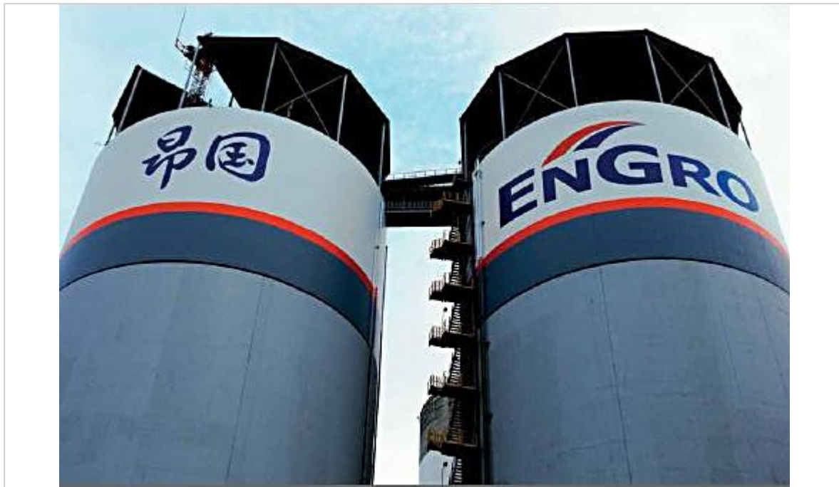
At Jurong Port, EnGro has two silos with a total storage capacity of 60,000 tonnes for specialty cement shipped in from its plants in China. Photo: annual report
