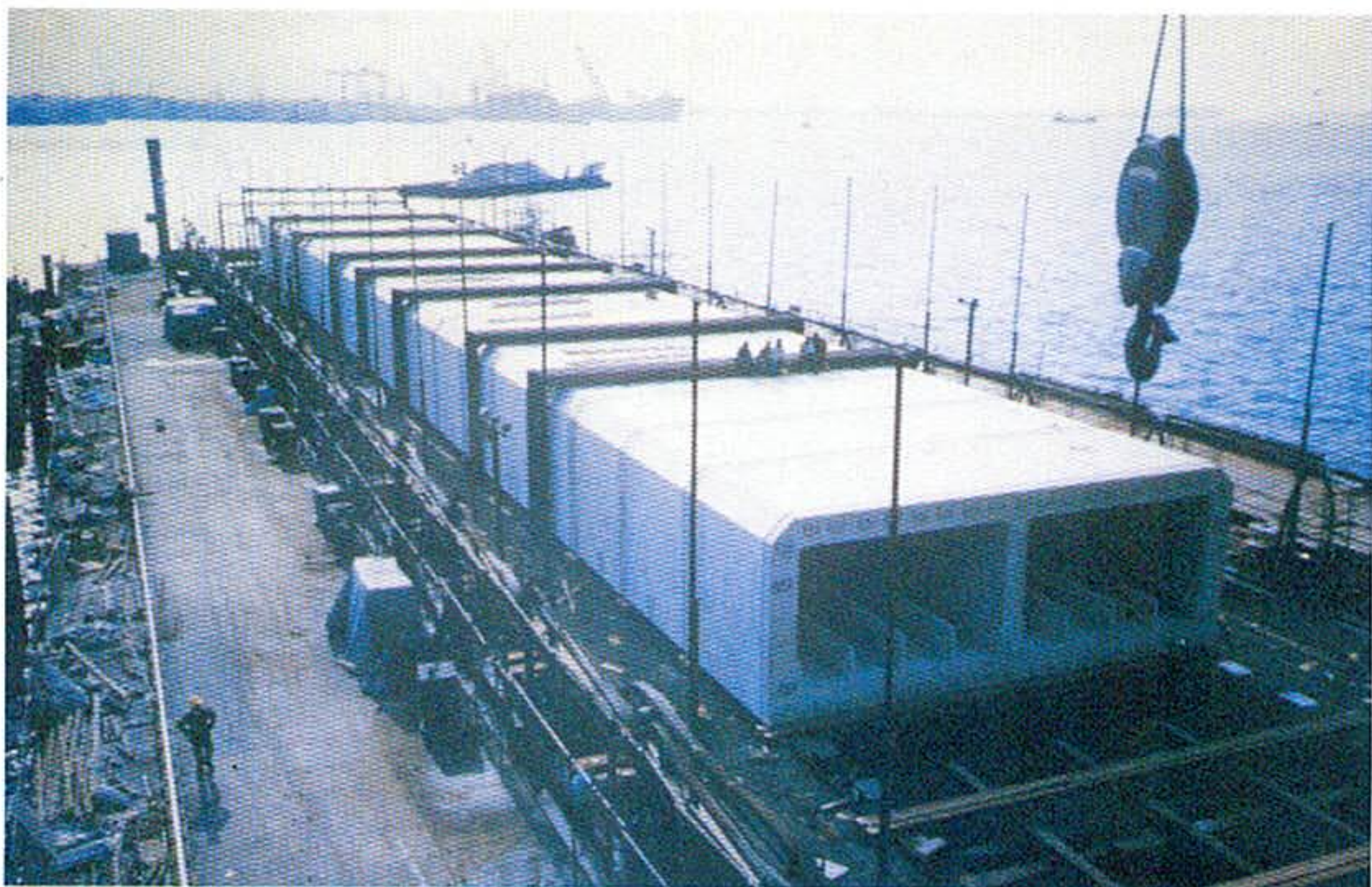
Picture 6: A close-up view of the aligned segments at the launching jetty
