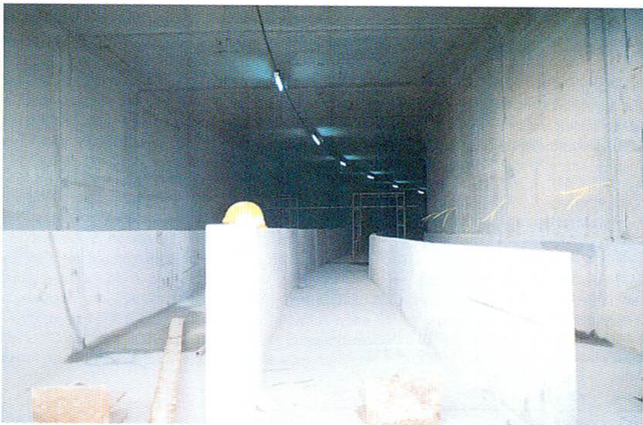
Picture 12: View of one side of the completed twin-box undersea cable tunnel
