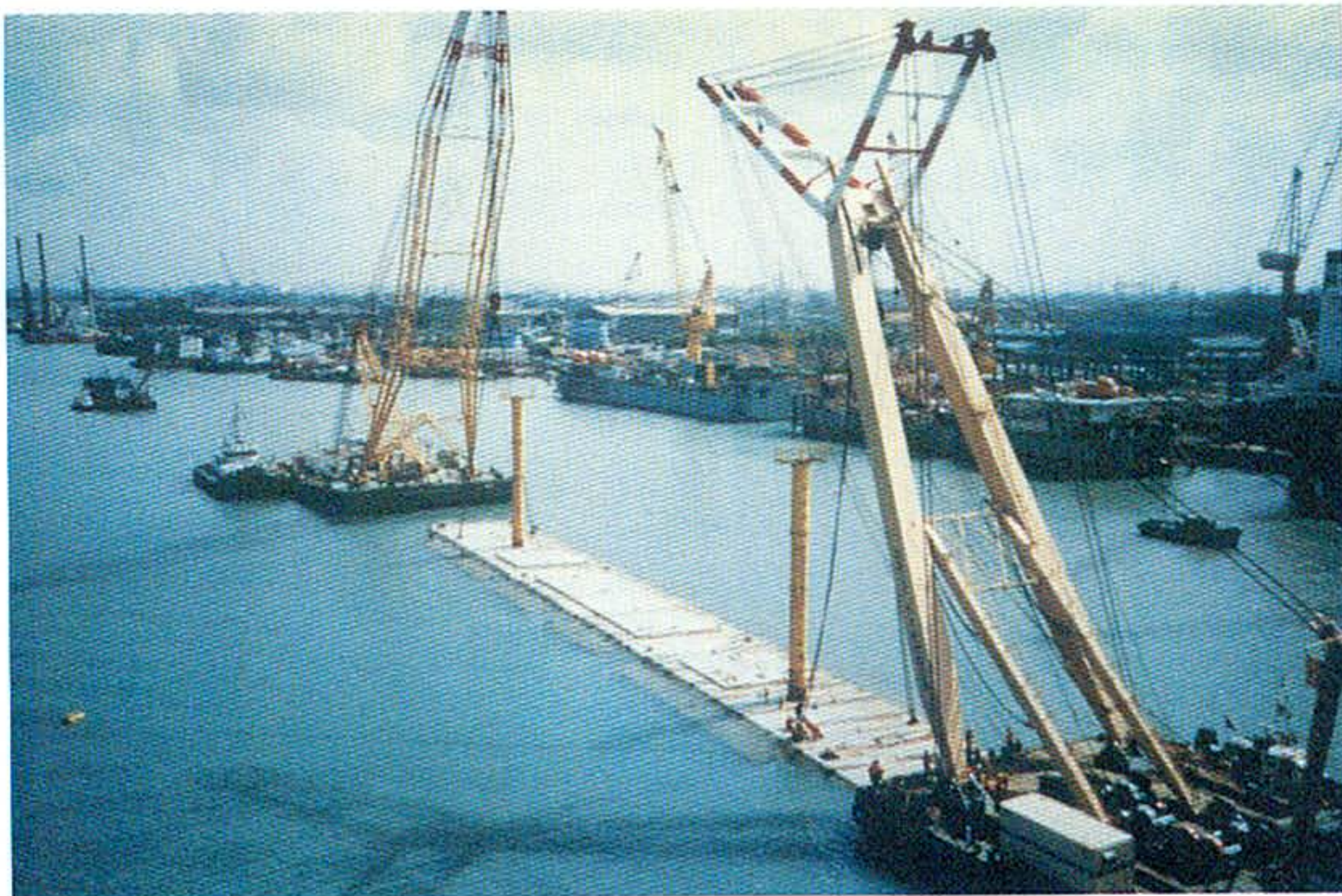
Picture 10: Sinking operation of tunnel element
