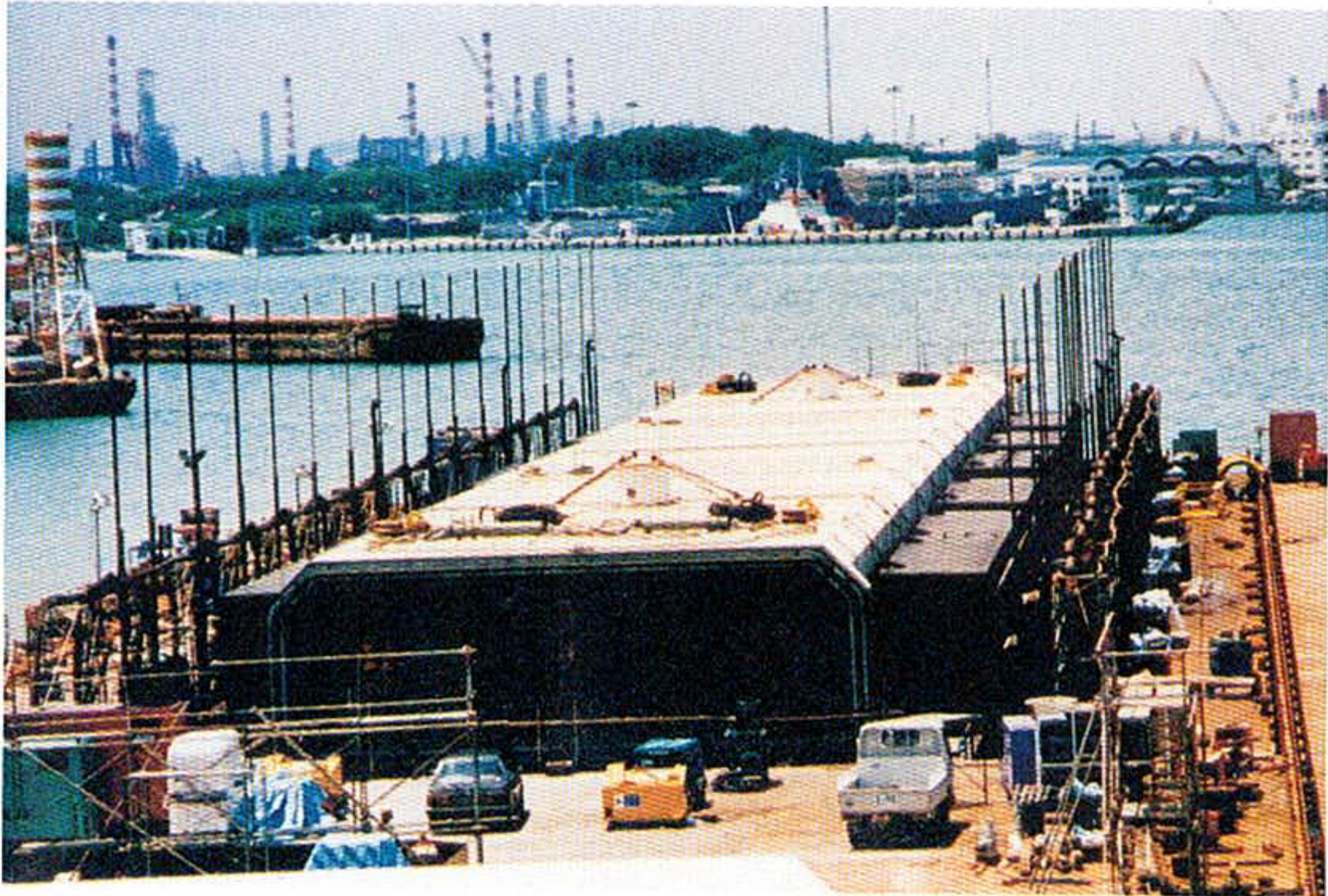
Picture 7: Each 100m element consists of 25 segments of 4m length
