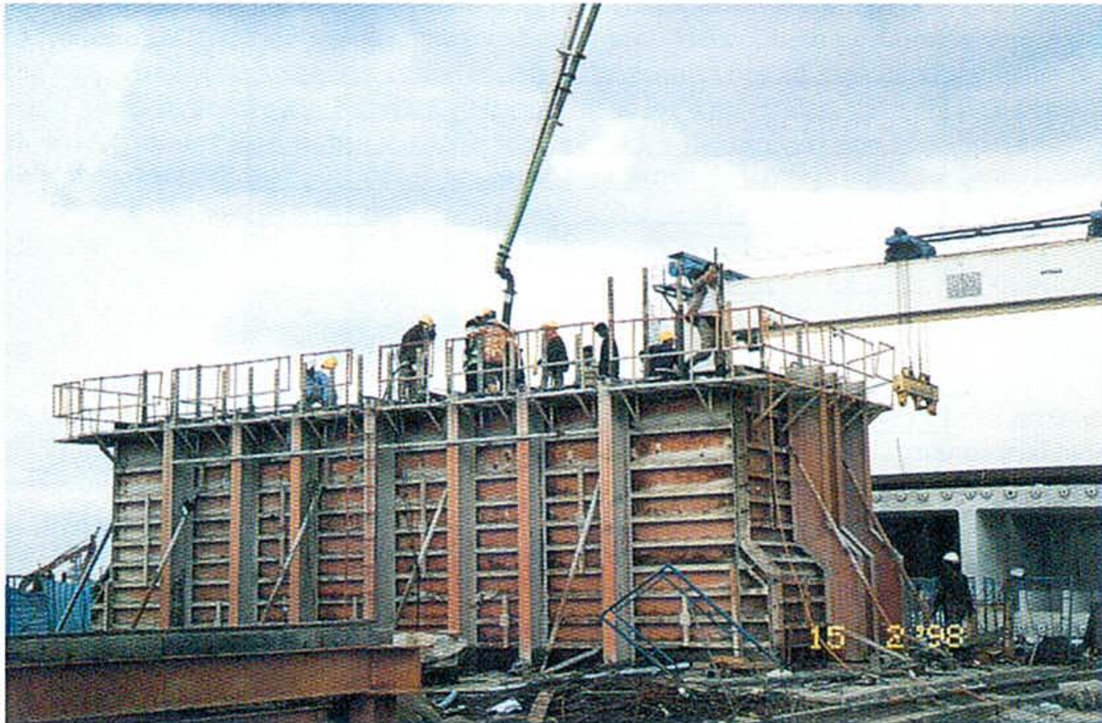
Picture 1: Casting of tunnel segment with SsangYong Cement's HSPBFC (Premium 4246) and S3 Technologies' integral waterproofer (SmartPruf)
