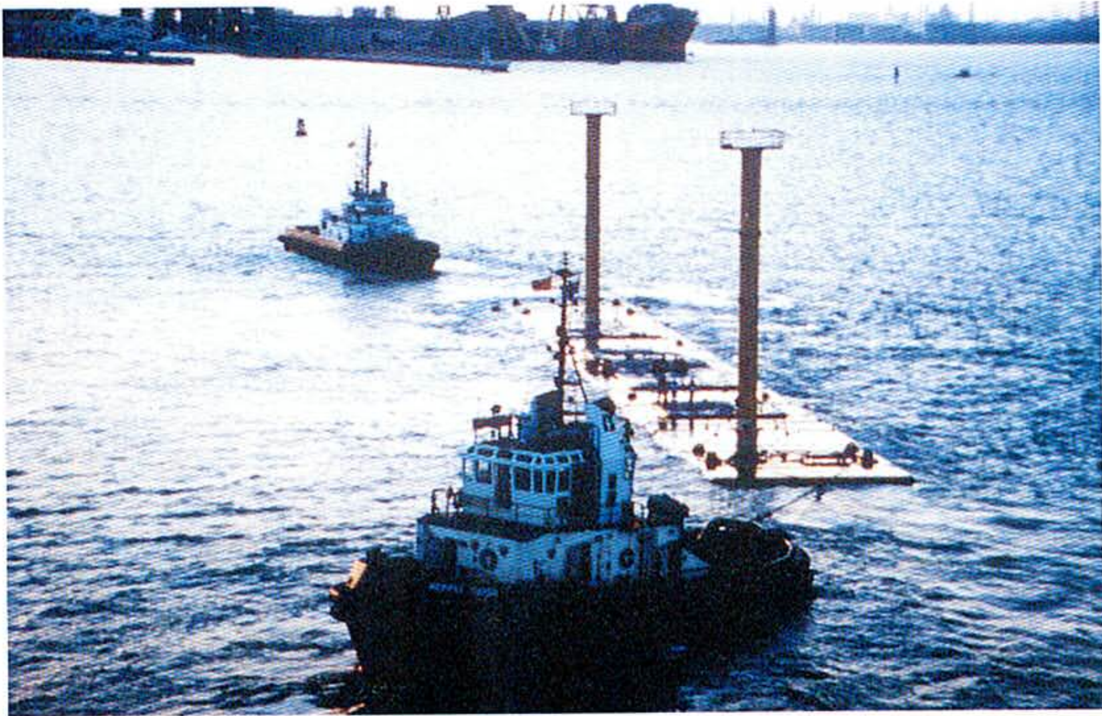
Picture 9: Towing of tunnel element out to its designated location
