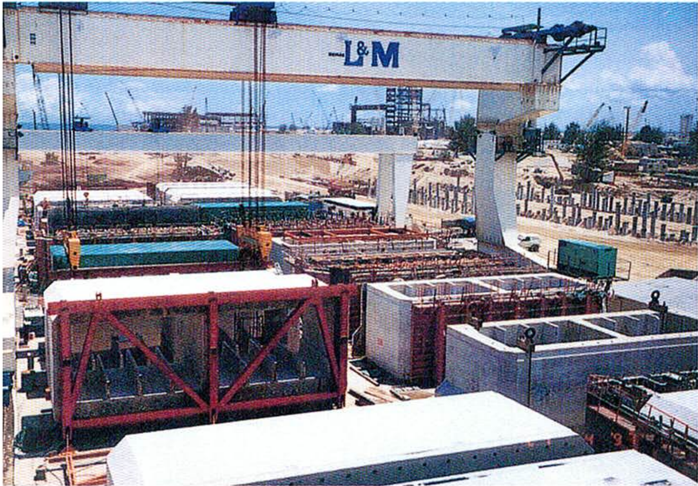
Picture 3: Precast yard for undersea tunnel segments
