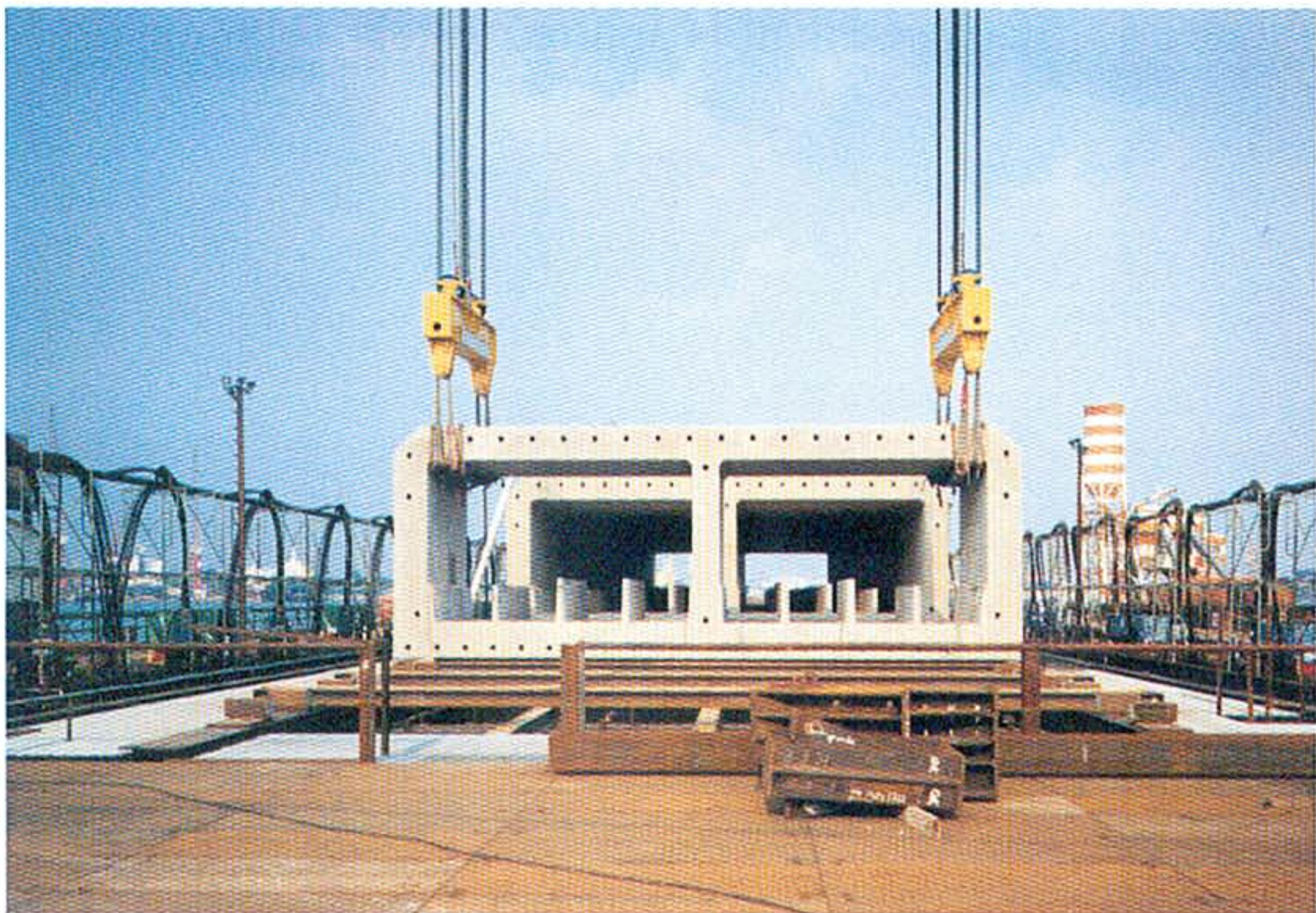
Picture 4: Precast segments are aligned at launching jetty
