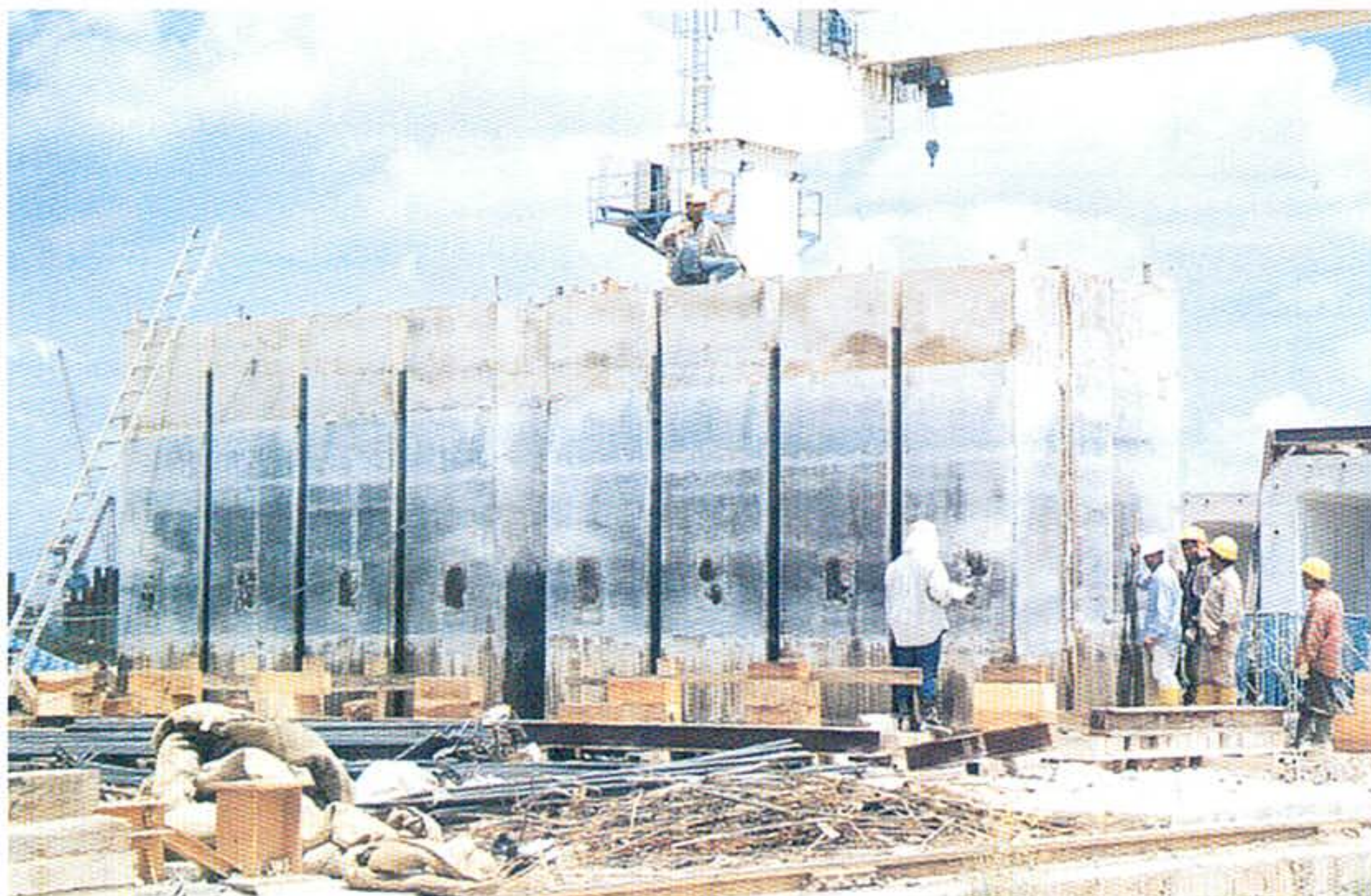
Picture 2: Rapid demoulding of tunnel segment after 24 hours
