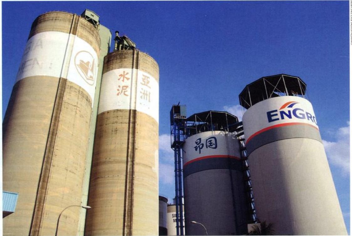
Cement is unloaded from ships and transferred to Engro's silo through conveyor belts and air slides at Jurong Port's cement terminal
